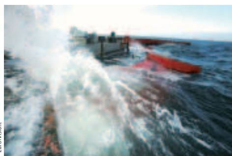
The Wave Dragon is a floating device consisting of two parabolic arms that reflects and enlarges waves towards a ramp. Wave energy is absorbed passively by overtopping water that is collected and short-term stored in a reservoir behind the ramp.
